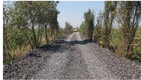
(b) Repaired causeway segment
